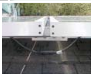
Right: MC connectors make series wiring easy.
